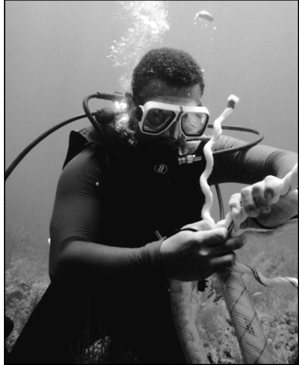
Figure 3-14. During the summer 1997 installation of reef mooring buoys in Guanaja, Bay Islands, Honduras, local diver Yovanni Bacca spliced lines underwater to attach the buoy line to the eyebolt on the ocean bottom. (Photo: Craig Quirolo)
